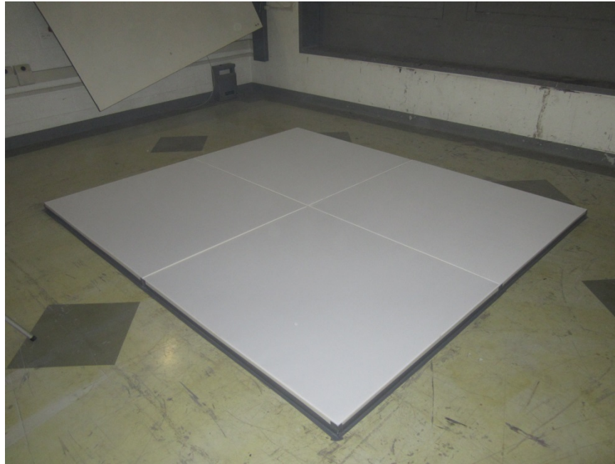
View of Installed Specimen
