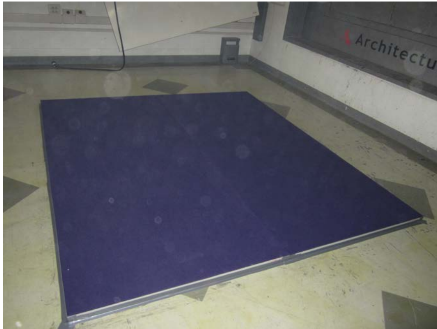
View of Installed Specimen
